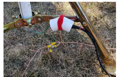
45 degree elbow helps protect chassis mount from shorting to poor weather
