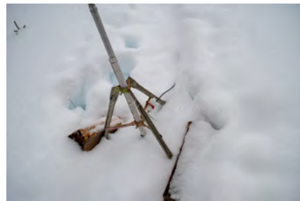
After a few inches of snow the feed point was buried! Two pieces of firewood help to prevent blow over
