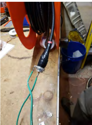
The SO-239 attached to feedline, sealed with electrical tape, two green wires go to antenna
